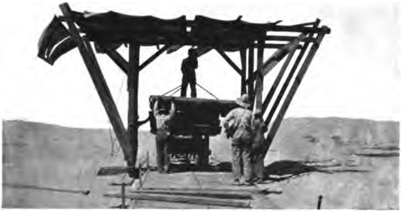
Unloading sections of plank road. Canopy protects workmen from sun.
